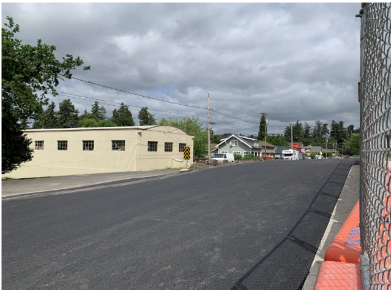
3 rd Street Paving
