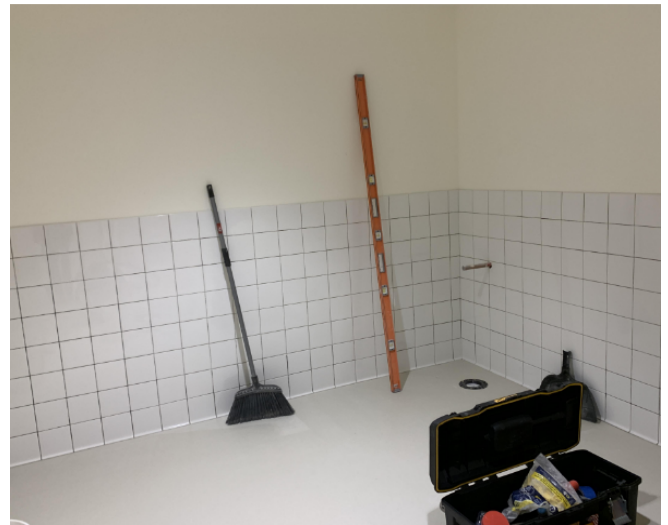
Level 1 Tile Installation
